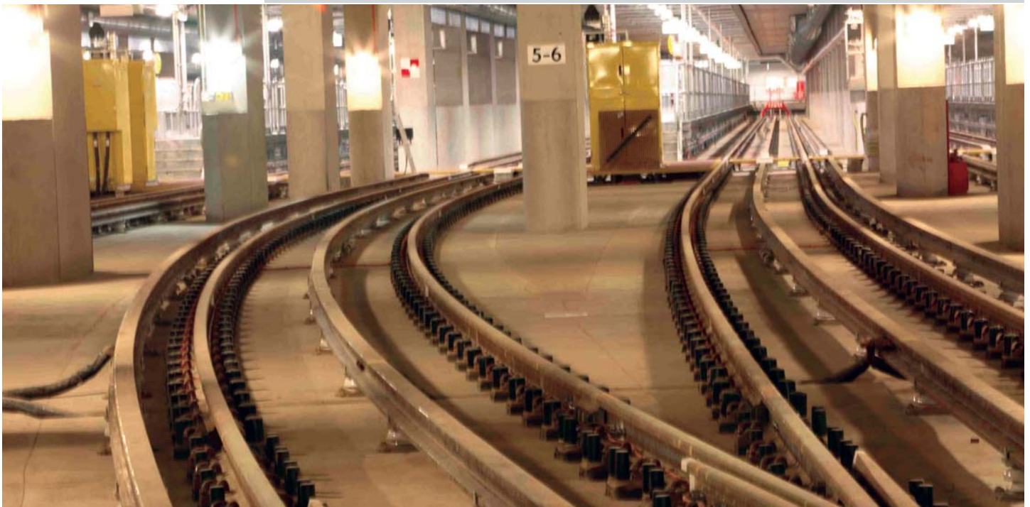
Part of the new 16 road London Underground Central Line Depot.
