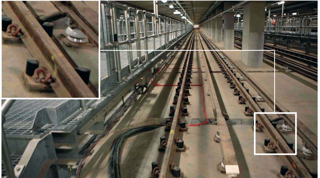
Hilti's Rail Anchors in use at White City.
