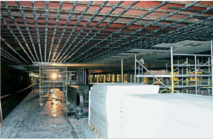
The metro managers in Prague have set high standards. New suspended ceilings must maintain in a fire for 90 minutes. Even the cable runs must have a high degree of fire resistance.
