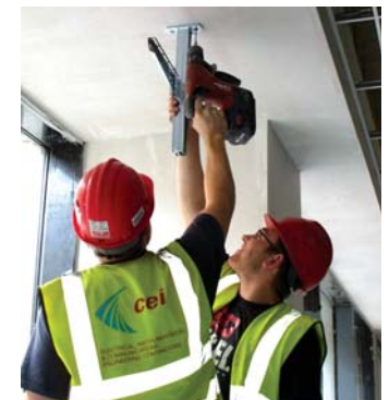
Labour efficiency improved by 25 per cent during installation.
